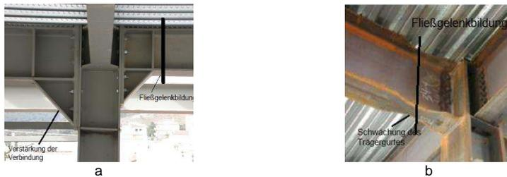
Figure 5: Constructive measures for the development of plastic hinges at the beam end
